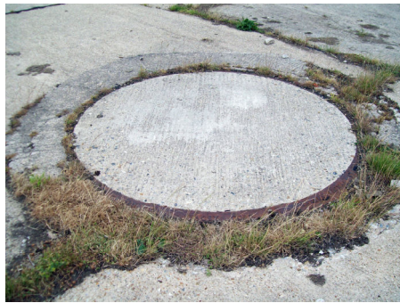
The manhole covers are still visible in2018.
