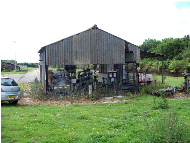
The pump for the Sculthorpe Pipeline.
